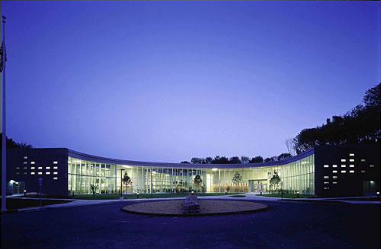
Burr Elementary School, Fairfield
